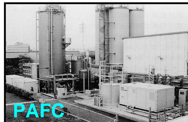
Sapporo Beer Co. Chiba (1999) 200kW PAFC by Toshiba/ONSI
