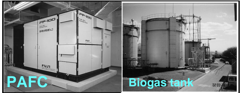
100kWx2 plants in Yamagata (2002) FujiElectric Co.
